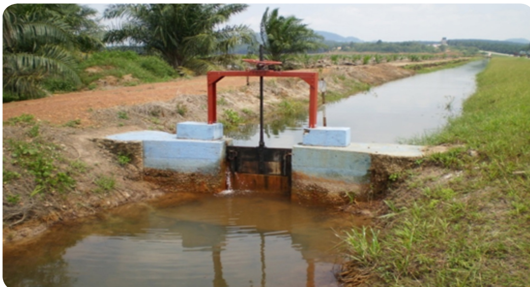
Photo 5 Watergate to control the watertable in an acid sulfate soil area in Malaysia
