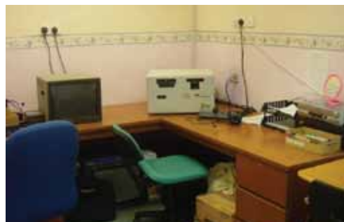
The video recording equipment room.
