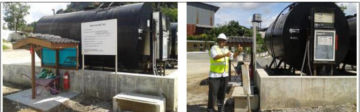
Diesel Skid Tank equipped with secondary containment, spill kit and oil & grease trap. Dispensing Hose stove inside containment.
