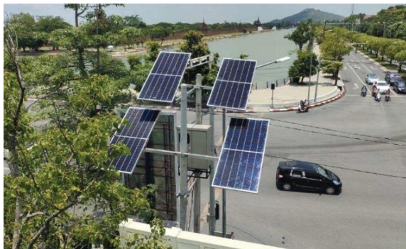
Exhibit 10: Solar System for the Traffic Lights at the Road Intersections © MCDC
