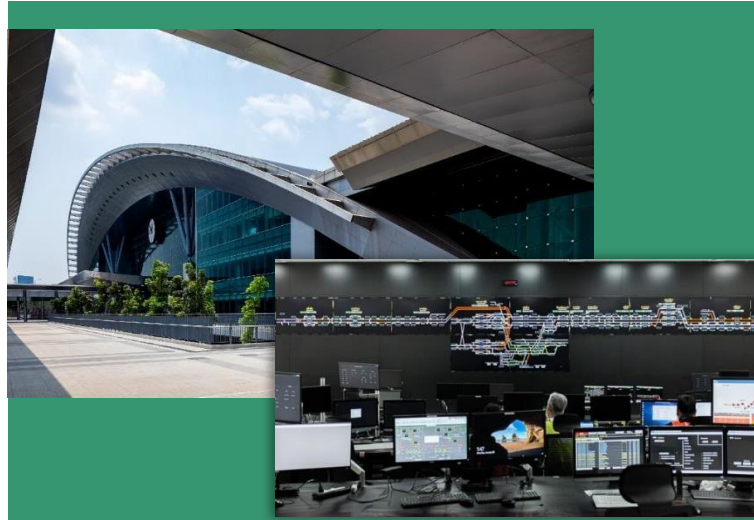
Exhibit 22: Operation control centre developed at Krung Thep Aphiwat Central Terminal Station to control and manage train operations. © SRT
